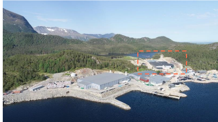
Norway - Nordheim commissioning
