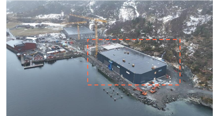
Norway - Haukå commissioning Q4-24
