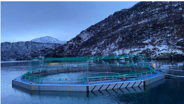
Norway - Closed Containment System
