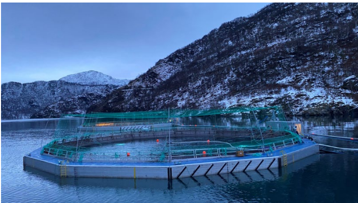
Norway - Closed Containment System
